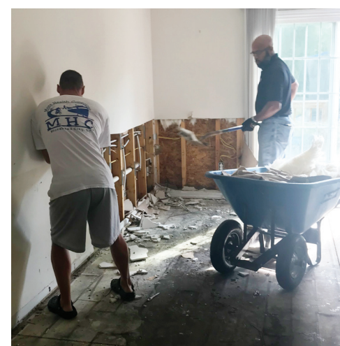
Volunteers from the NALC Disaster Relief Foundation tear out drenched drywall in a North Carolina letter carrier’s home after Hurricane Florence had receded.
