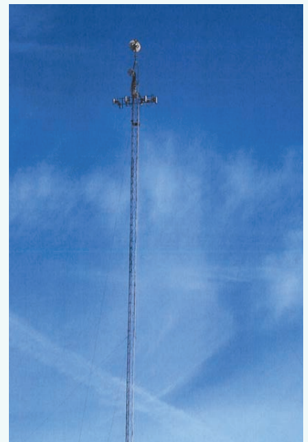
Nalcrest's Wi-Fi tower
